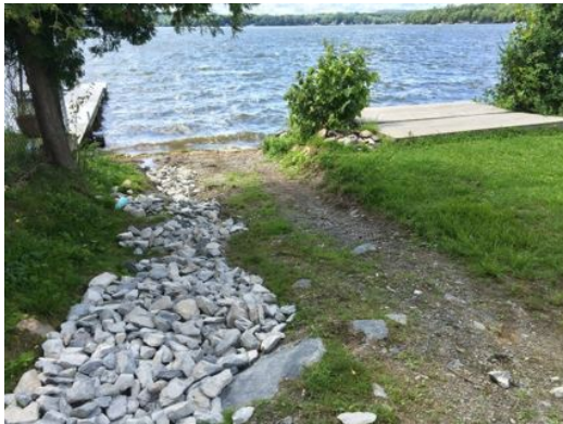
Lakeshore path stabilized with stone to prevent further erosion
