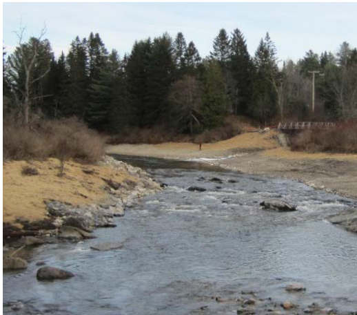
After removal of the East Burke Dam on the East Branch of the Passumpsic River
