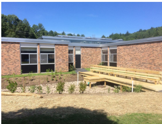
Completed construction of bioretention area with boardwalk
