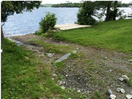
Eroding path leading to lakeshore
